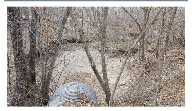
Recent, unvegetated ditch maintenance activity and insufficient buffer left some ditch channels susceptible to erosion and sedimentation.
